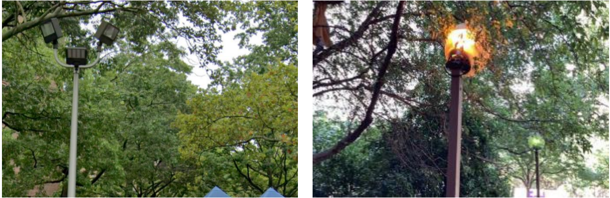
Figure 38 Typical Site Lighting
