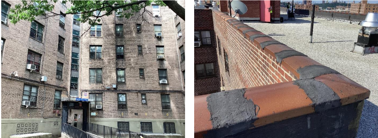
Figure 20 Typical Building Exterior ( left ), Parapet and Roof ( right )
