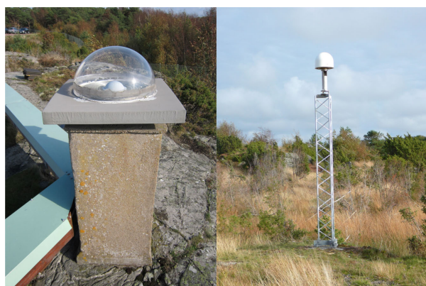
Fig. 5 The pillar and antenna of the IGS station ONSA (left), and the mast and antenna of the IGS station ONS1 (right).
