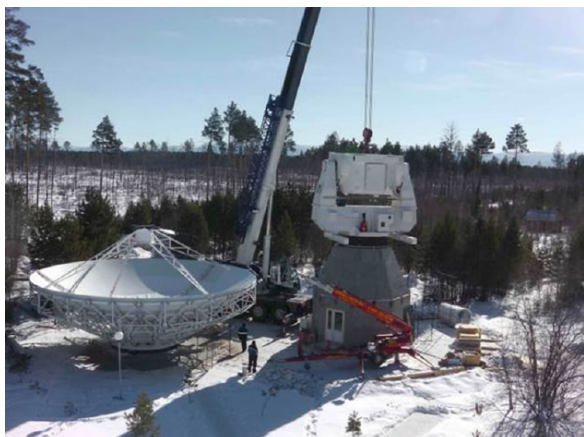
Fig. 3 On-site installation works.
