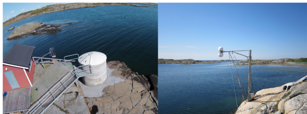
Fig. 7 The traditional tide gauge (left) equipped with a radar and several bubbler sensors in the well, and the GNSS-R based tide gauge (right).
