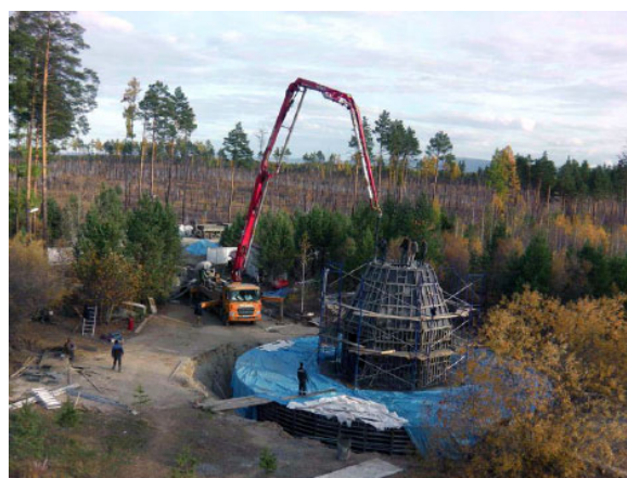
Fig. 2 Antenna tower construction.
