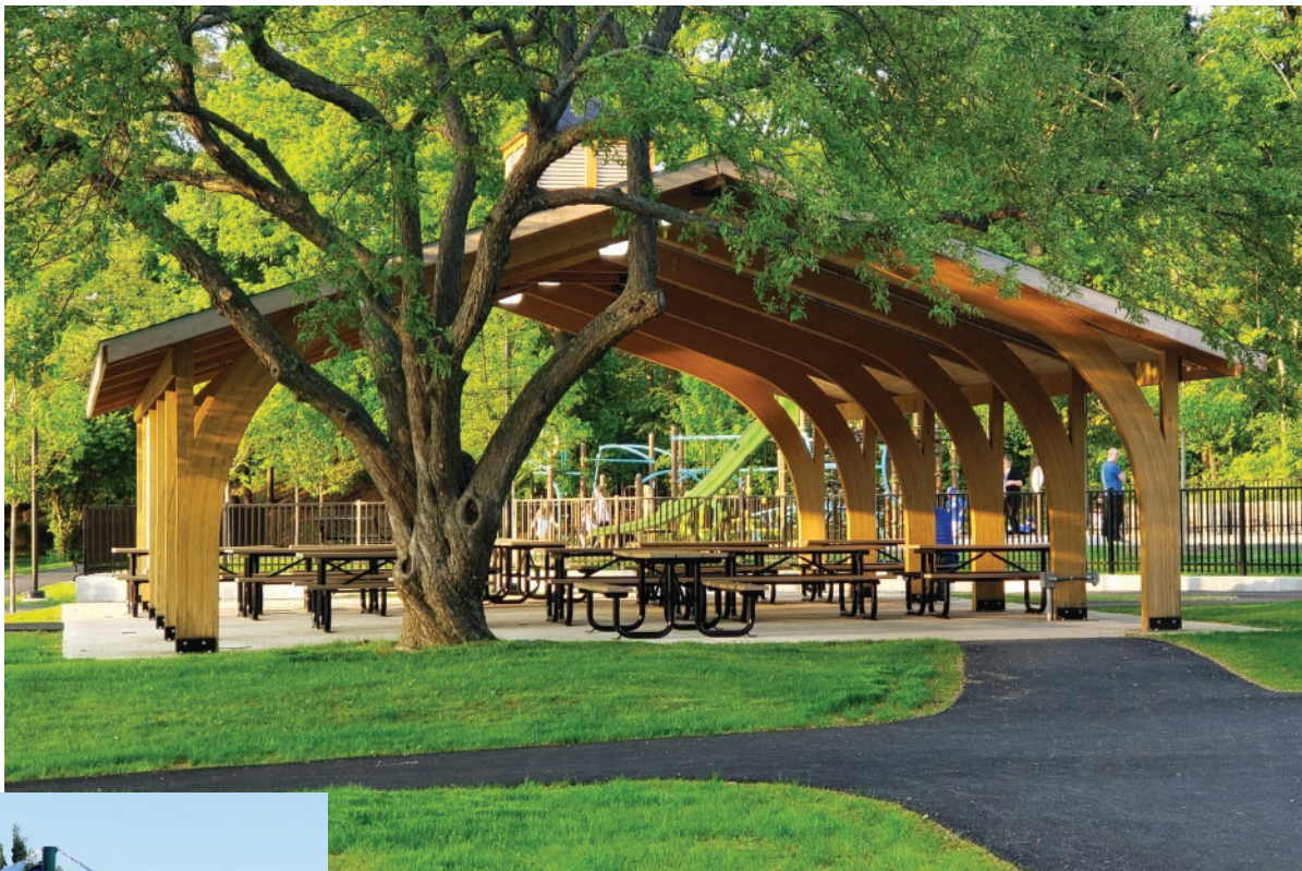
Wood structures can include laminated beams, tongue-and-groove sub-roofs and a variety of roofing materials from shingles to standing seam metal.
