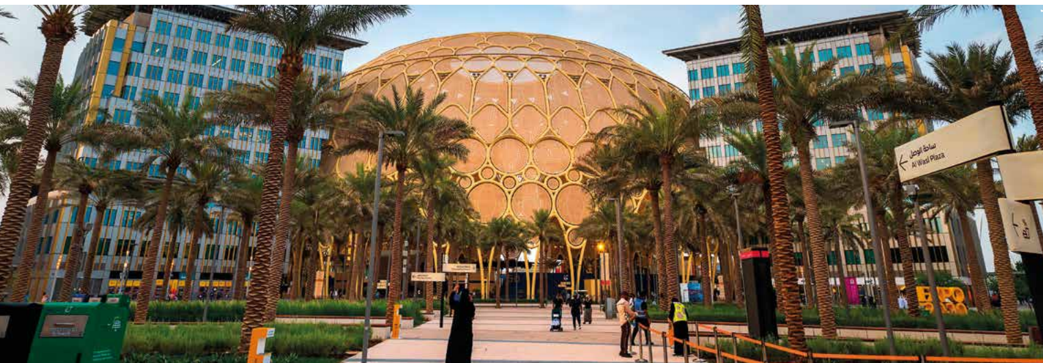
Al Wasl Plaza dome at the Expo 2020 in Dubai is the central hub for the exposition.
