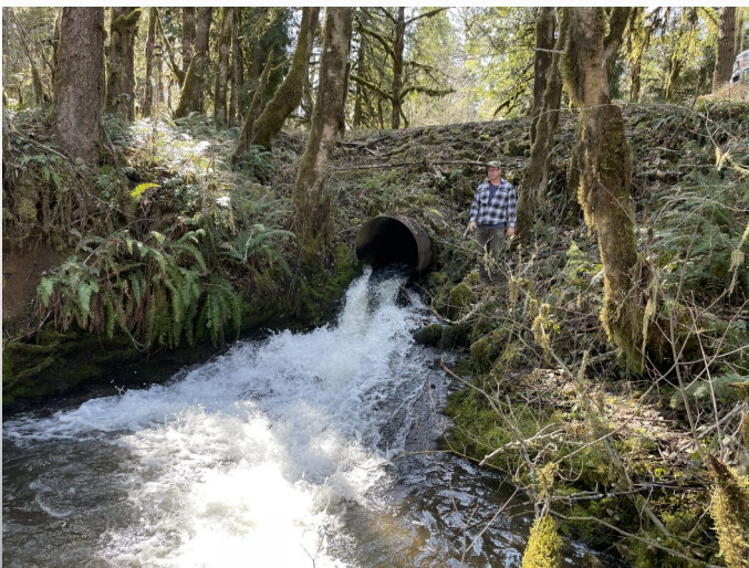
Steve Kendall standing next to a culvert slated for replacement.
