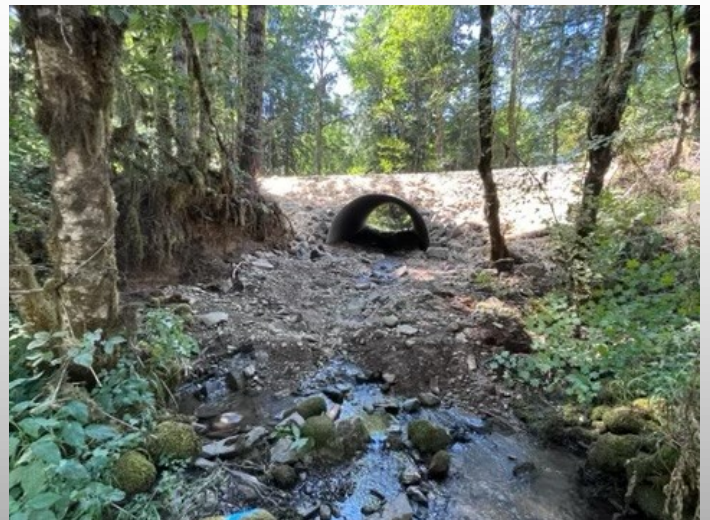
Completed fish passage after culvert replacement.
