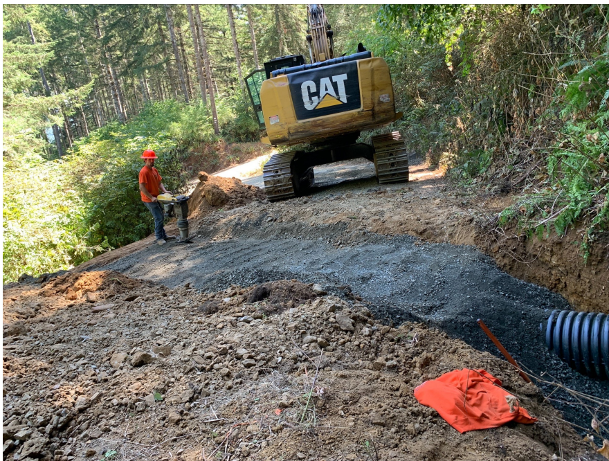
Culvert being installed at Low Incline Timber Sale.
