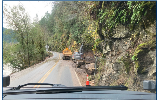
ODOT Co-op clearing the road of a slide
