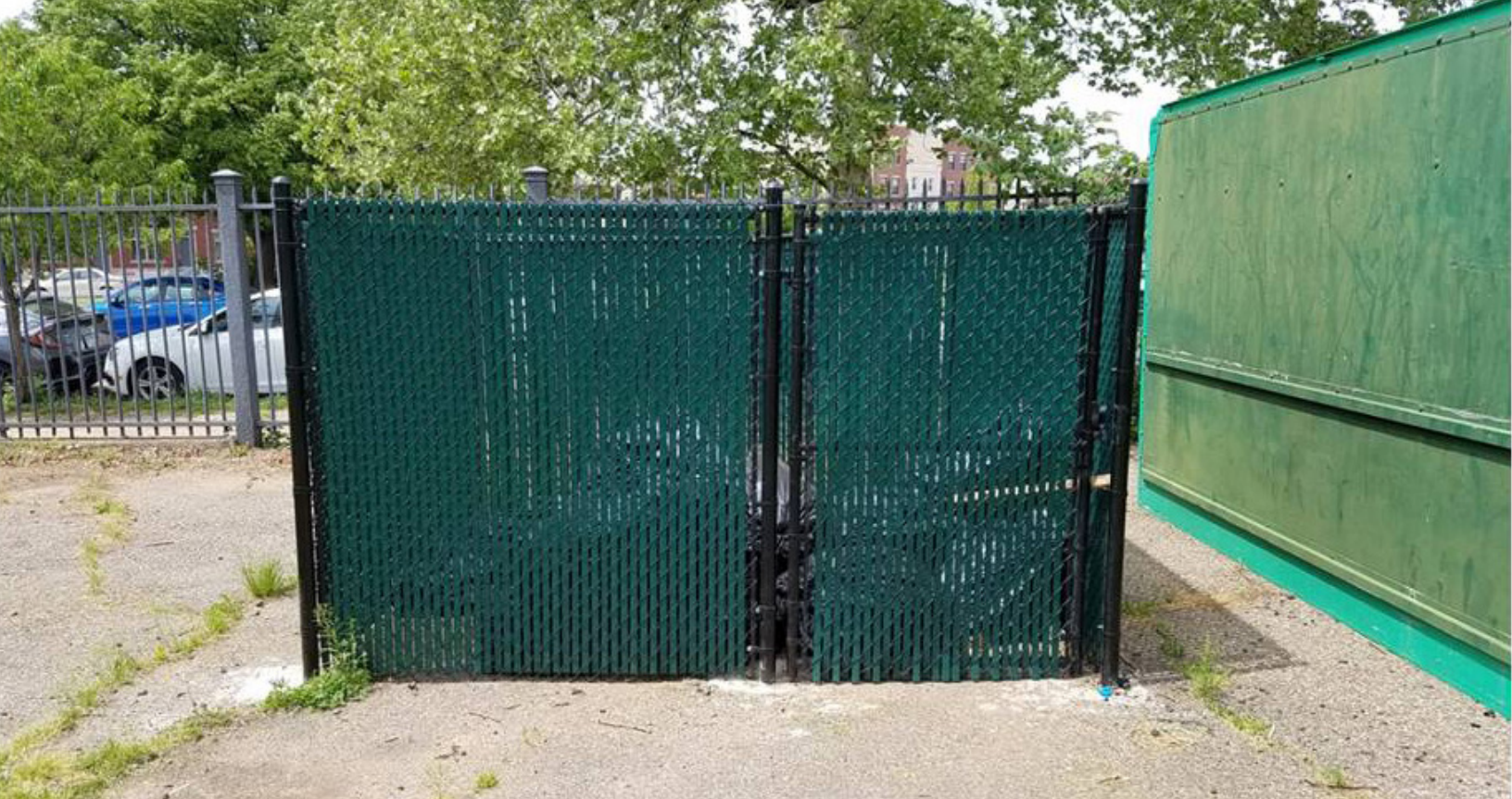
Waste corral installed by Philadelphia Parks & Recreation
