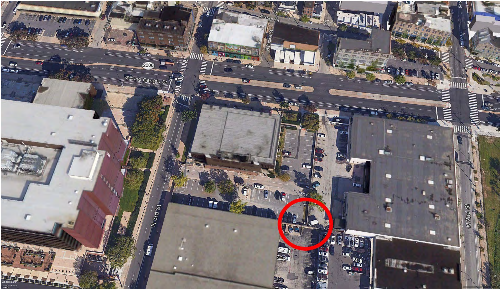
Figure 13 – FAB North Aerial View
