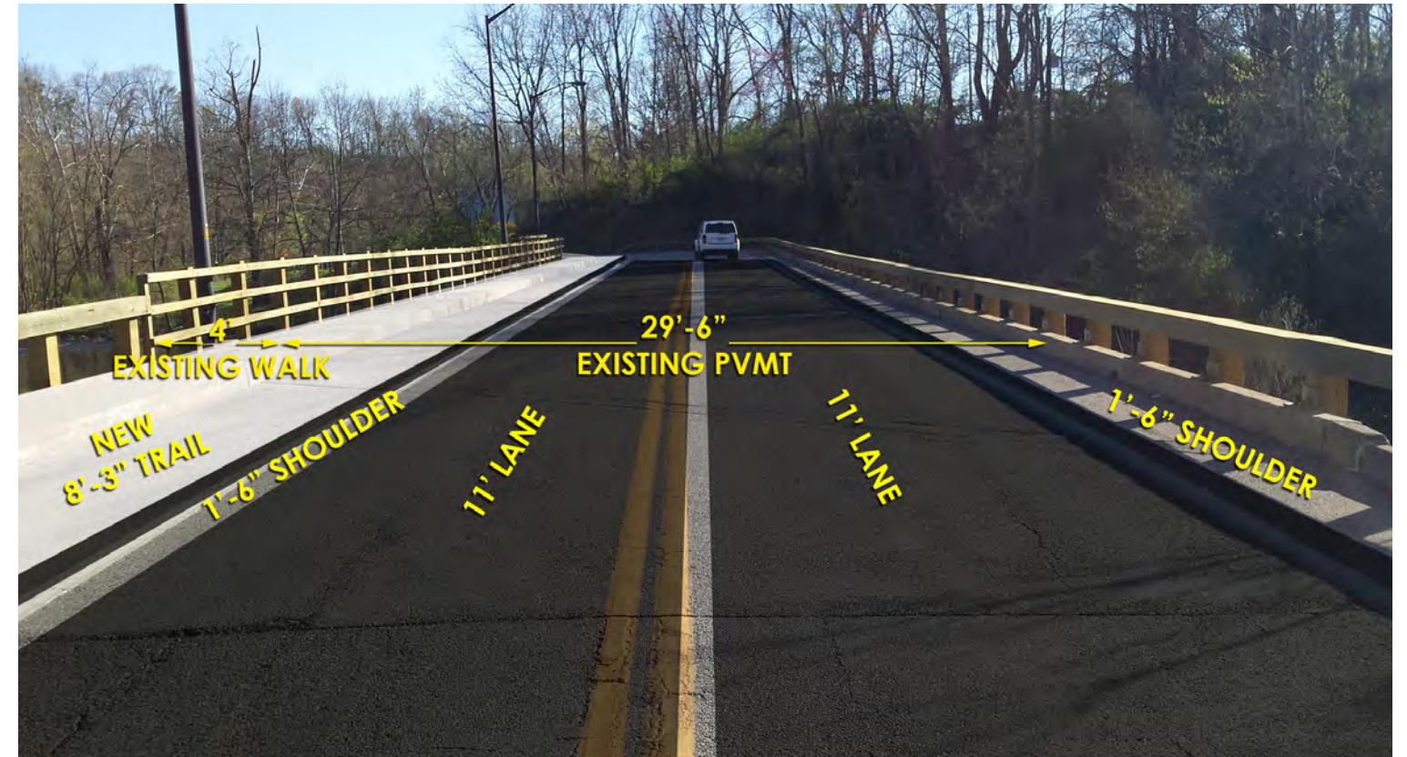
Mason Mill Bridge
