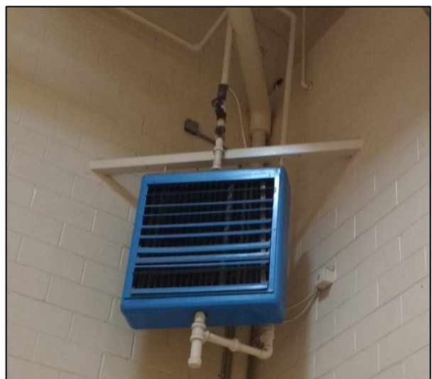
Hot Water Unit Heater (Typ. of 4)
