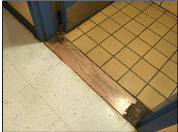
Corridor & Toilet Room Flooring
