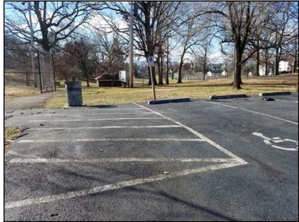
Handicapped Accessible Parking Spot
