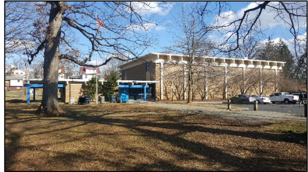
Exterior Masonry Walls
