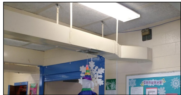
Exposed Ducting
