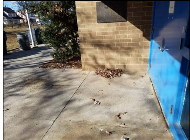
Sidewalk at Main Entry Doors
