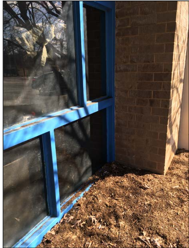
Hollow Metal Frames with Single Pane Glass
