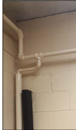
Interior CMU walls
