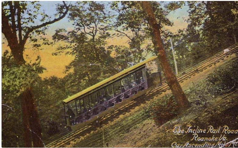
Figure 17. Side view of the incline
