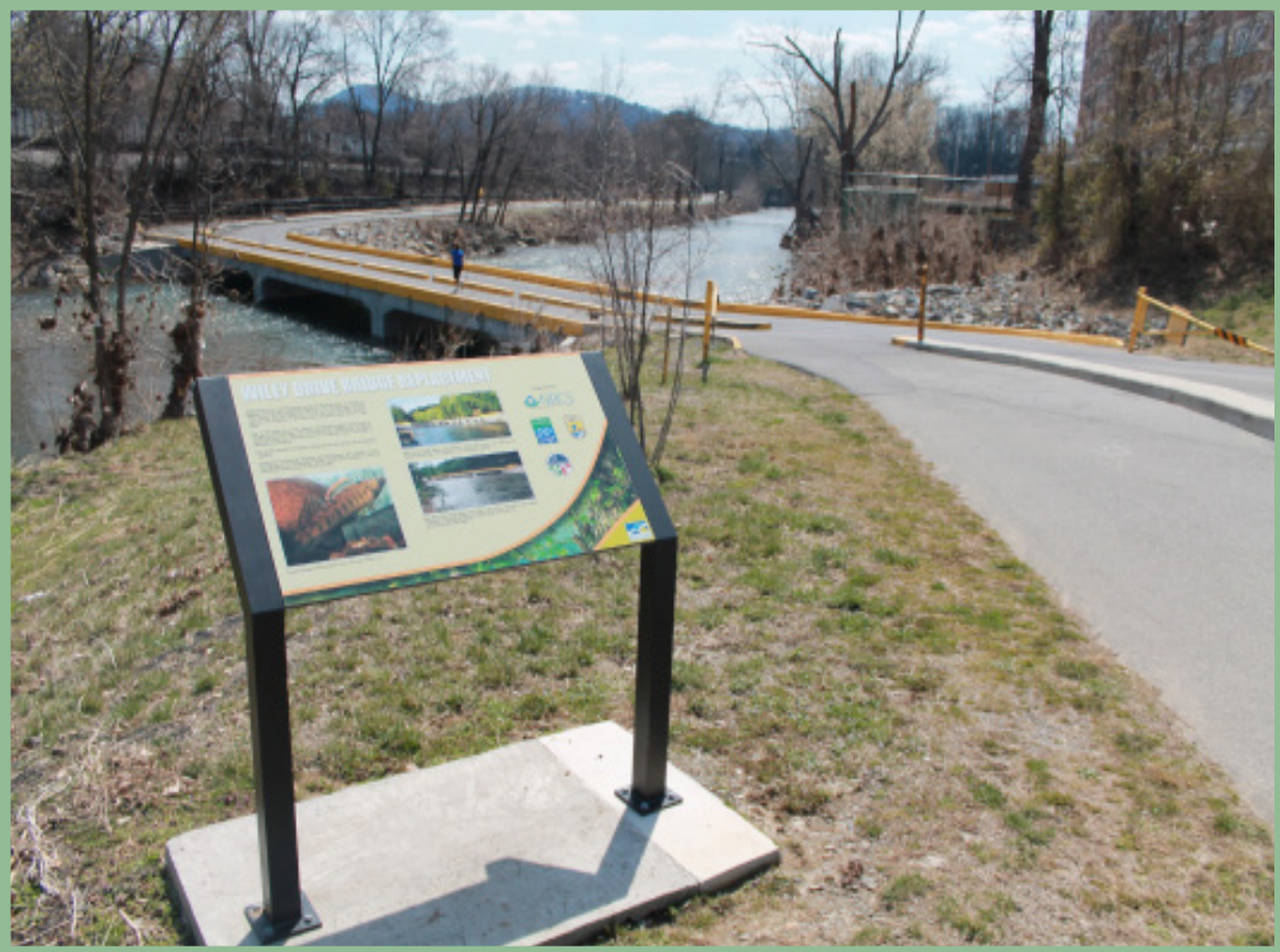
Installed historic marker for Wiley Bridge Replacement on Roanoke River Greenway
