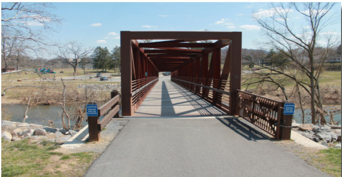
Roanoke River Greenway, Bridge approaching Vic Thomas Park
