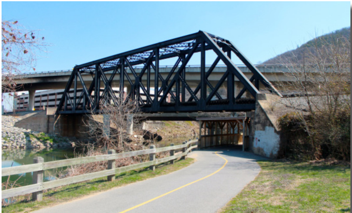
'Railroad Bridge,' near Carillion Hospital
