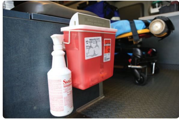
Fig. 2-10: Biohazard containers, such as those used for sharps disposal, are one type of engineering control.
