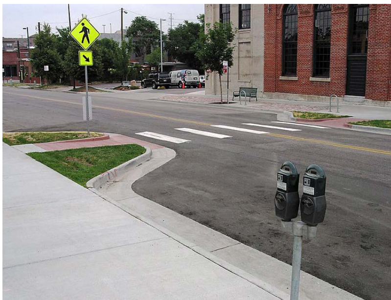
Bus Stop in Parking lane after Pedestrian Curb Extension (Vancouver, BC)
