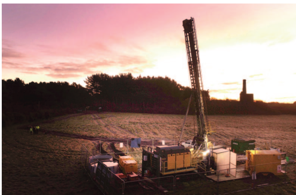
Exploration drilling for geothermal waters – United Downs 2019
