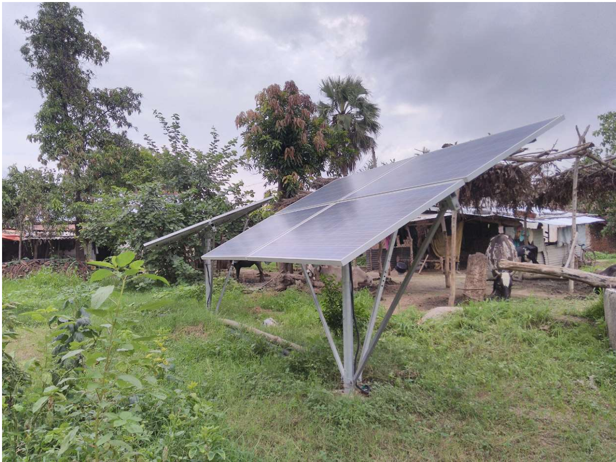
Figure 3: Solar pump-set in a SEWA member's field in Anand District, Gujarat
