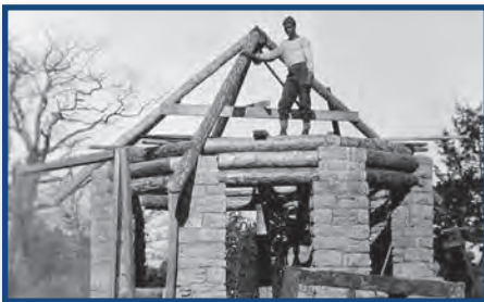
Stonemason from Company 1743 of the Civilian Conservation Corps, building a structure at Washington State Park in the 1930s.
