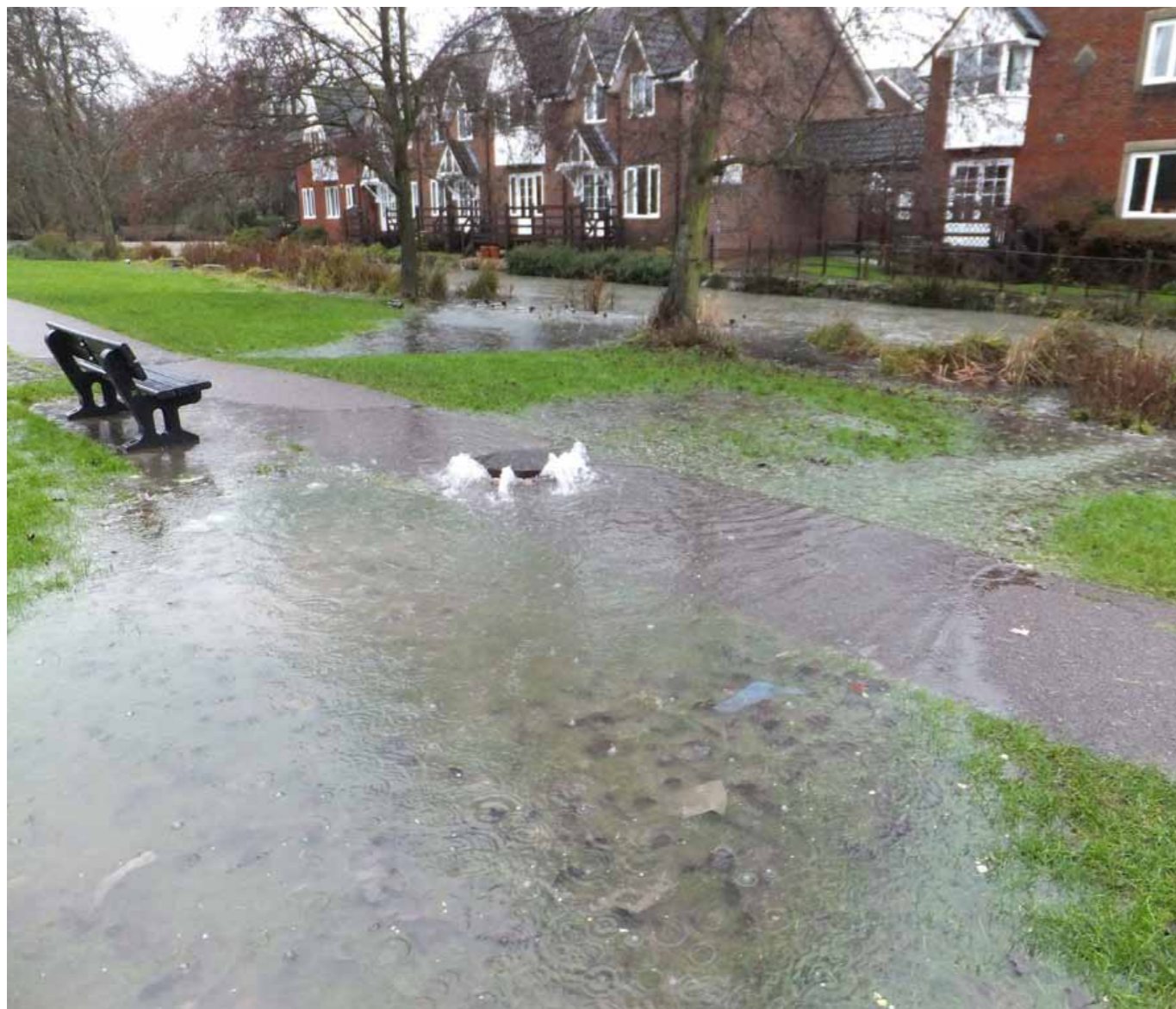
▲ Figure 1. When surface water sewers surcharge the results can sometimes be very dramatic! (© Gerrald Isaaman)
