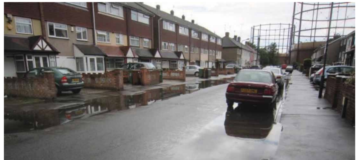
▲ Figure 6. Streets with no green or permeable areas are an all-too-common sight. Water has no option but to pond until there is available capacity in the drainage system. (© Wilhelmina Drayton)
