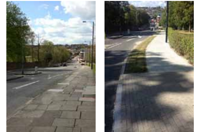
▲ Figure 5. There are opportunities to increase infiltration everywhere. The introduction of this green verge, designed with additional storage in the subbase to allow more water to be accommodated, improves the urban environment, reduces diffuse pollution and reduces flood risk. (Source: from Owen Davies)
