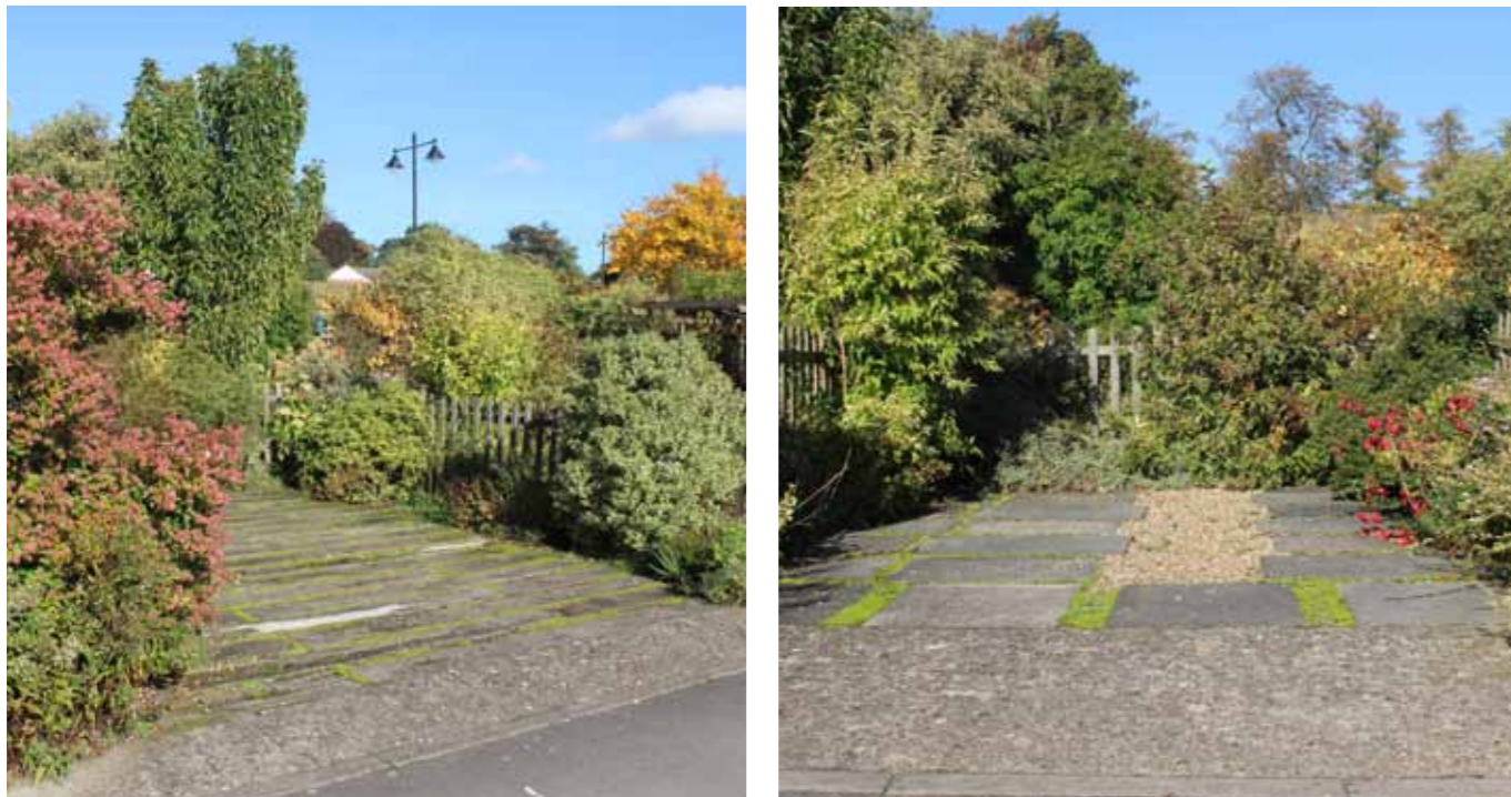
▲ Figure 7. Vehicles can still be parked on these very attractive front gardens, but they are permeable, reducing the burden on traditional drainage systems. (© Robert Smith)
