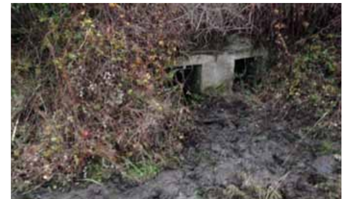
▲ Figure 4. Siddington Meadows taking water away from the village down the natural flood plain after four road under drains had been unblocked — a simple act by a landowner that helped to reduce flood risk to the village flooding and improved ecological status for both meadow and water quality. (© Jenny Phelps)
