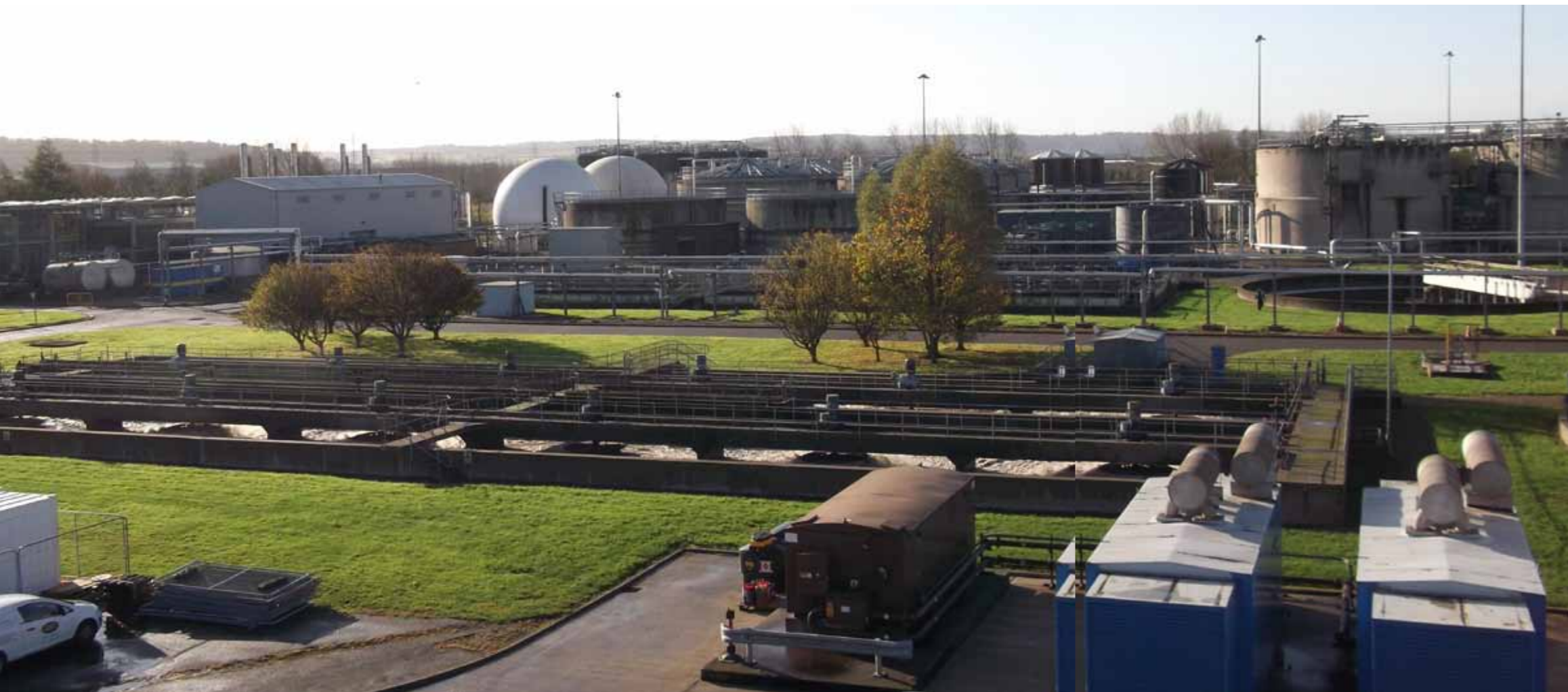
▼ Figure 3. Avonmouth Wastewater Treatment Works: beyond the ‘engineering paradigm’. (© Chad Staddon)
