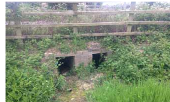
▲ Figure 4. Siddington Meadows taking water away from the village down the natural flood plain after four road under drains had been unblocked — a simple act by a landowner that helped to reduce flood risk to the village flooding and improved ecological status for both meadow and water quality. (© Jenny Phelps)
