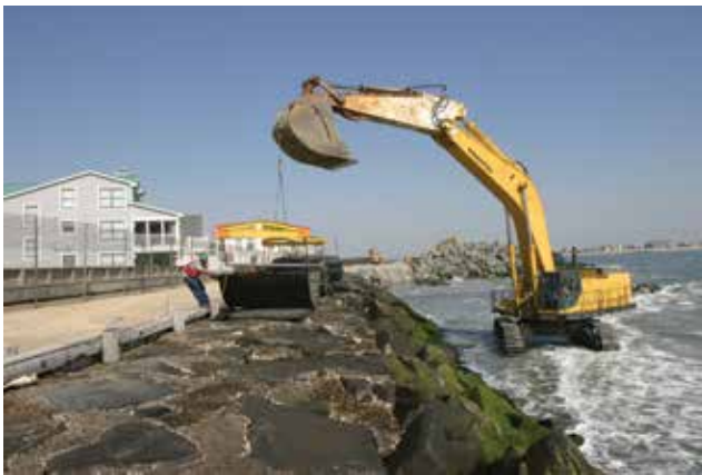
A seawall is constructed in New Jersey by the US Army Corps of Engineers. The hard defensive measures that are widely deployed today were typically built to dampen storm surge and limit erosion, not keep out normal but higher tides.
