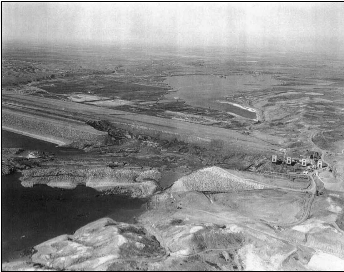
Figure 6-17: Gravel and stone facing can be seen in the material that slid away from the upstream embankment at Fort Peck Dam on September 22, 1938. Source: Records of the U.S. Army Corps of Engineers, Record Group 77, National Archives and Records Administration, College Park, Maryland.
