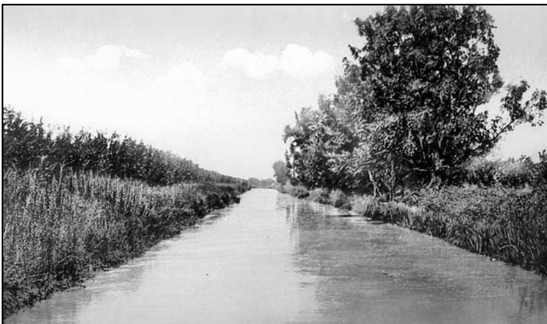
Figure 7-3: An irrigation canal in the San Joaquin Valley about 1900. Source: Donald C. Jackson postcard collection.
