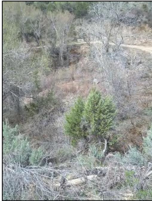
Photo 3. Existing siphon, view southwest from point of siphon intake (Photo 2). Drain grate is visible along with Leroux Creek.
