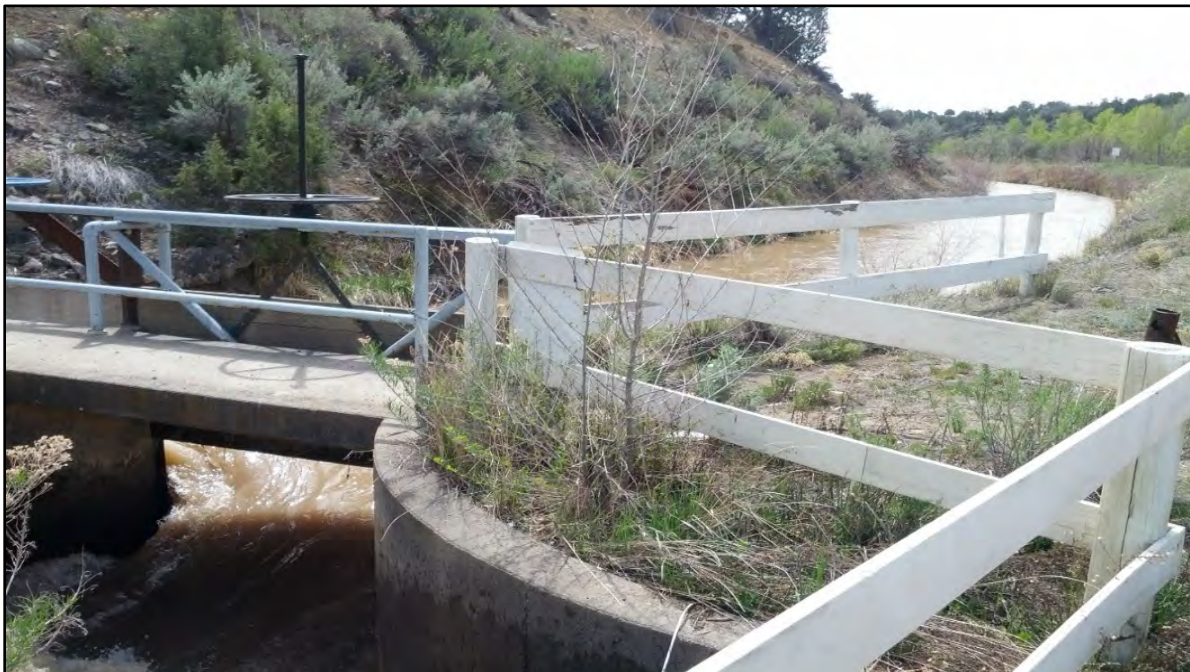
Photo 2. Existing siphon intake, view east, after water has entered the canal.
