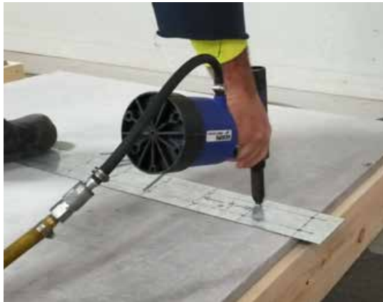
A pneumatic setting tool is used to install the peel rivets.
