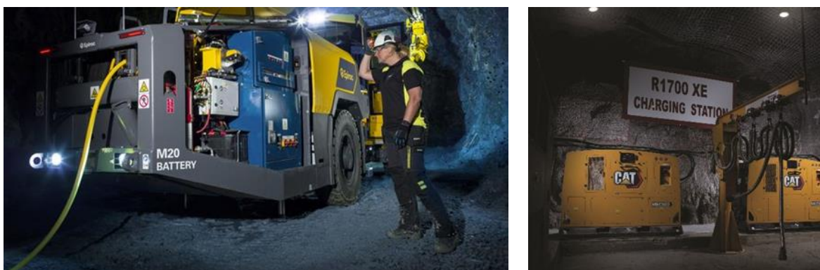
Figure 3-2: Battery charging via power cable (left, source: Epiroc) and example of a charging station (right, source: Caterpillar)
