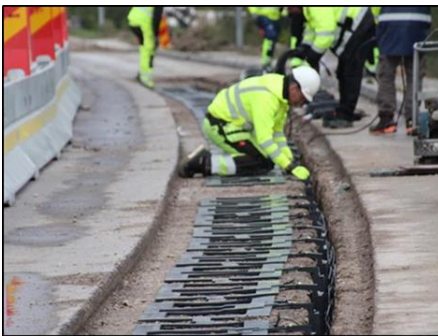
Figure 3-5: Induction coil in the ground [13]
