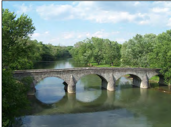
Photo 6: Wilson Bridge spanning Conococheague Creek
