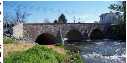
Garis Shop Road Bridge
