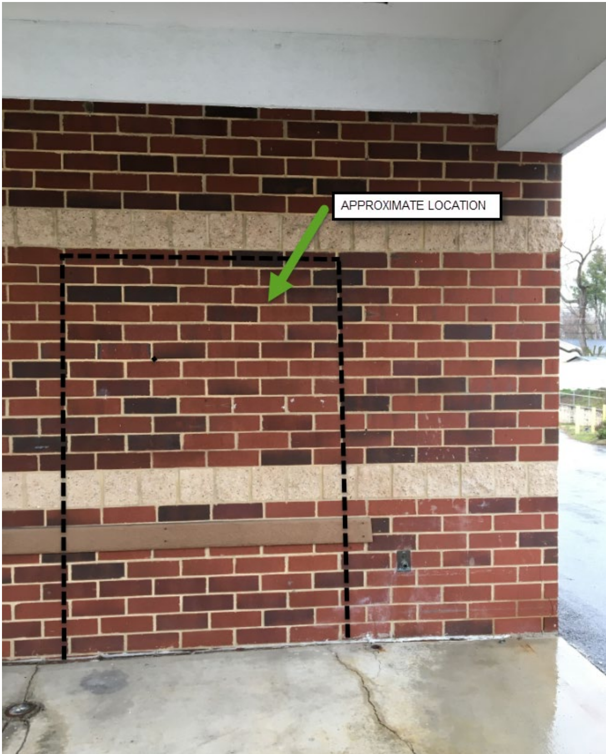
Front of Building
