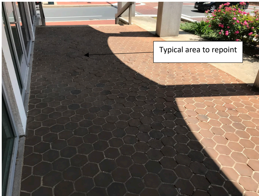
County Administrative Building: Hexagonal Brick Repointing
