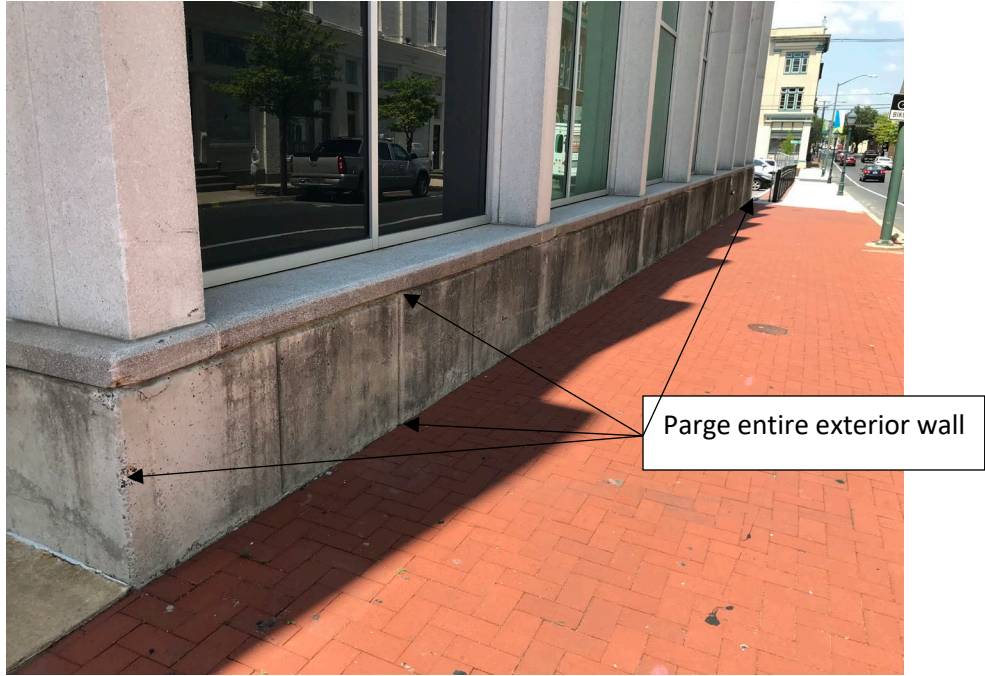
County Administrative Building: Wall Foundation to Parge
