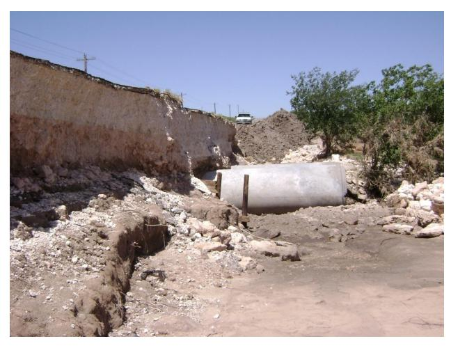
Water washed out the downstream side of F.M. road 759 at the south fork of the Wolf Creek, 3 miles east of State Highway 70.
