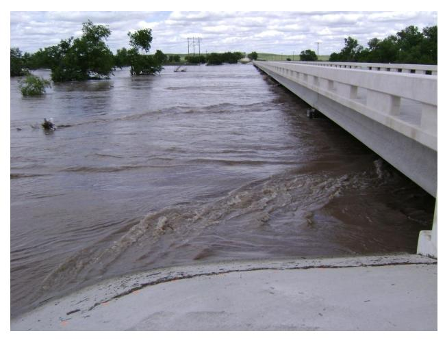
Wolf Creek at the Texas State highway 305 bridge at Lipscomb. Looking north along the upstream side of the bridge. Note the high water mark on the bridge abutment.
